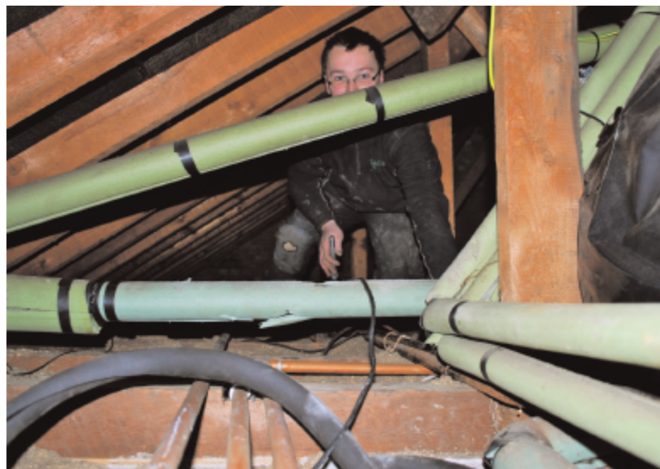
CPHS installer Krystian in the loft when fitting the flue
